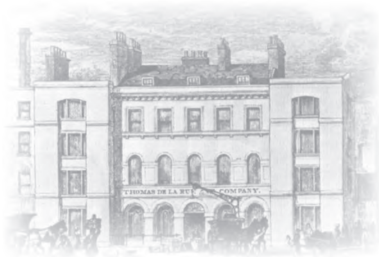
The office of De La Rue and Company
